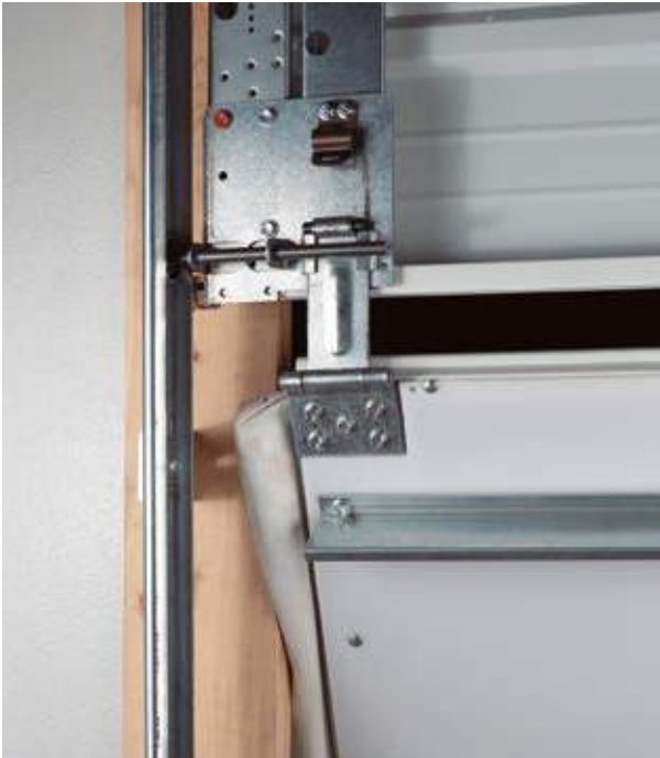
Inside View of Single Bottom Section
